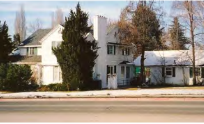
Moved Office and Shelter
